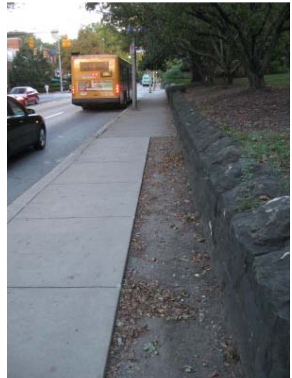
Photo 5 - An area along Fifth near Morewood Avenue with a recently constructed sidewalk far below standards.
