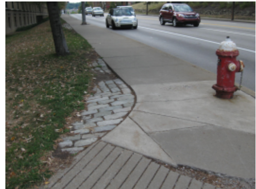
Photo 4 - Northeast corner of Morewood at Forbes Avenue. The landing area for wheelchair occurs over block stone and grass. The block stone is utilized in numerous places along Forbes Avenue in an attempt to widen pedestrian pathways. The area settles and subsequently becomes filled with silt and standing water during rains and ice in freezing weather.
