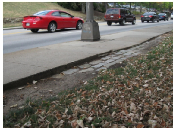
Photo 8 - A buffer or tree lawn here would eliminate the need for pedestrians to move around this light pole along Forbes Avenue near Beeler Street. Settlement of the block stone here approaches 6 inches.
